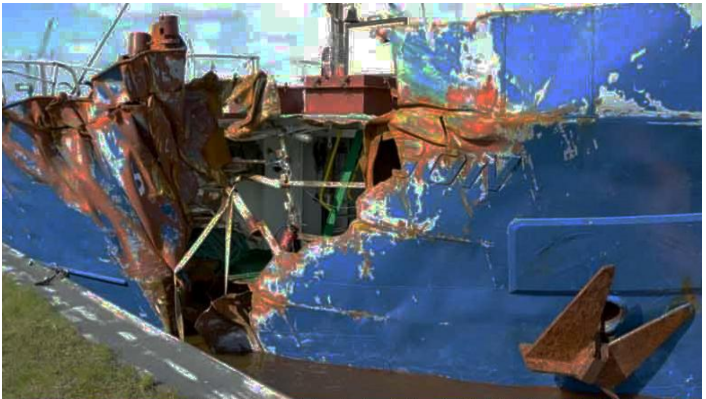
In the area of the starboard side of the forecastle there is a three by five meter hole / Photo: Wasserschutzpolizei
